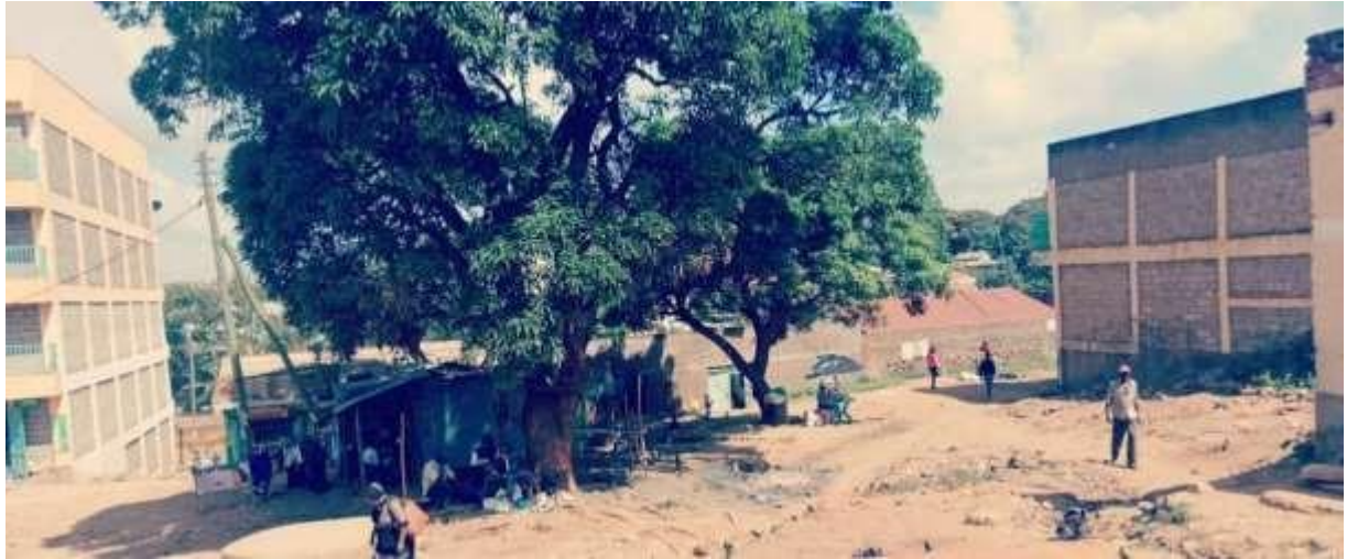
Plate 12: High density residential buildings along the corridor proposed for improvement
