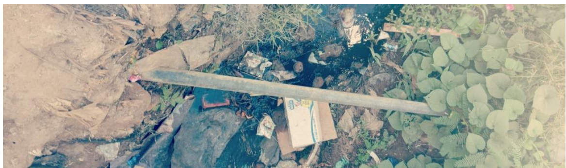
Plate 5: One of the water pipeline across the corridor to be improved
