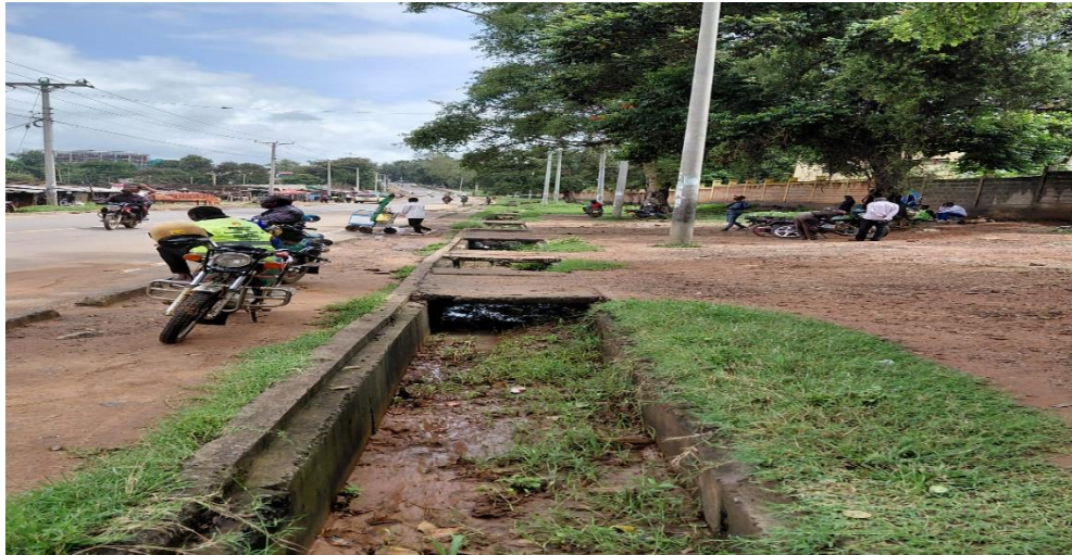
Plate 6: The existing drainage along the corridor proposed for improvement
