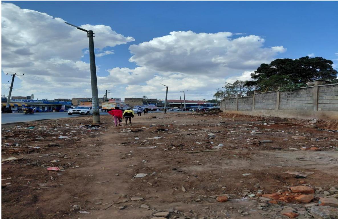
Plate 11: A section of the road corridor which is rocky
